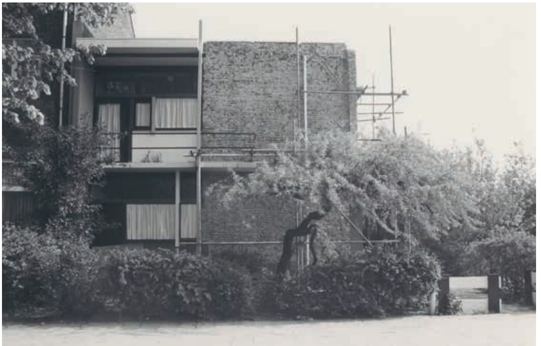
6. The bare brickwork of the wall on Prins Hendriklaan in 1979. On the wall below the window of Rietveld's former studio (bottom left) render is still visible (Bertus Mulder archive)
