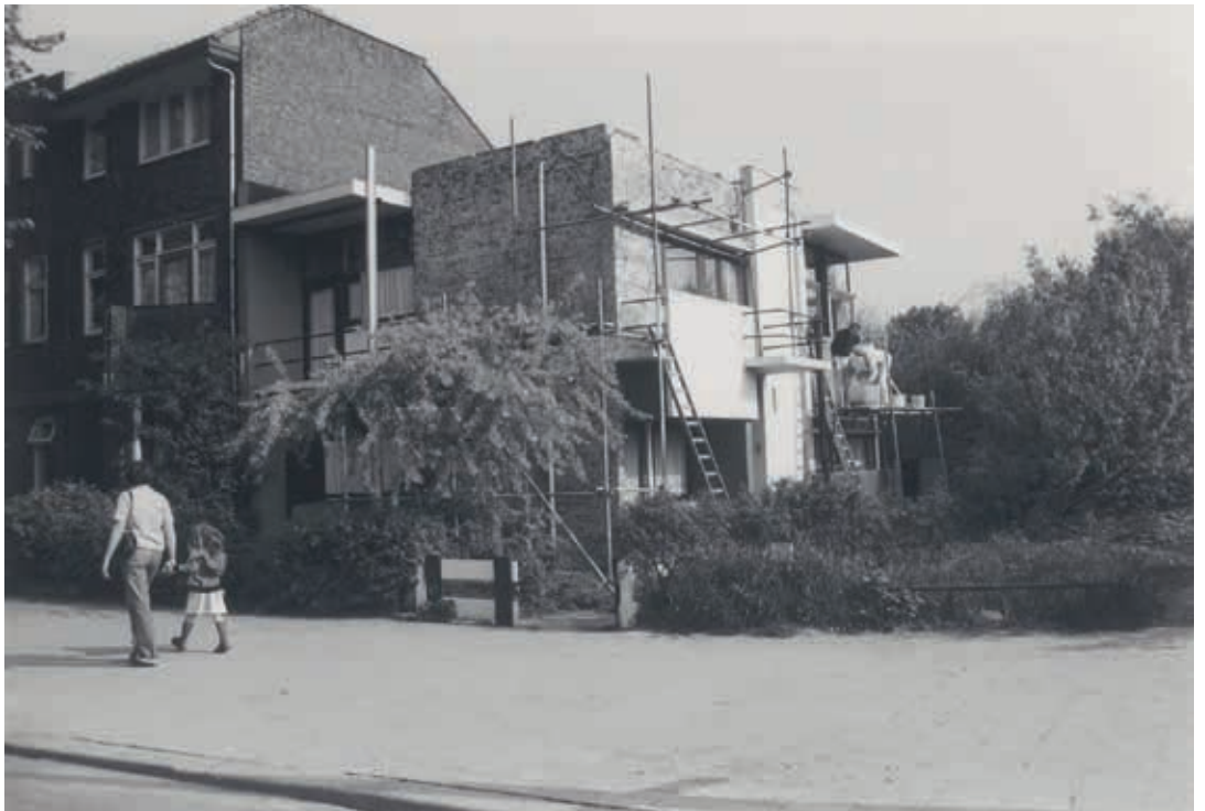
5. In 1979 the Rietveld Schröder House was once again scaffolded after the reappearance of the problems with the plasterwork. Large areas of render were first chipped away, after which a new coat was applied (Bertus Mulder archive)
