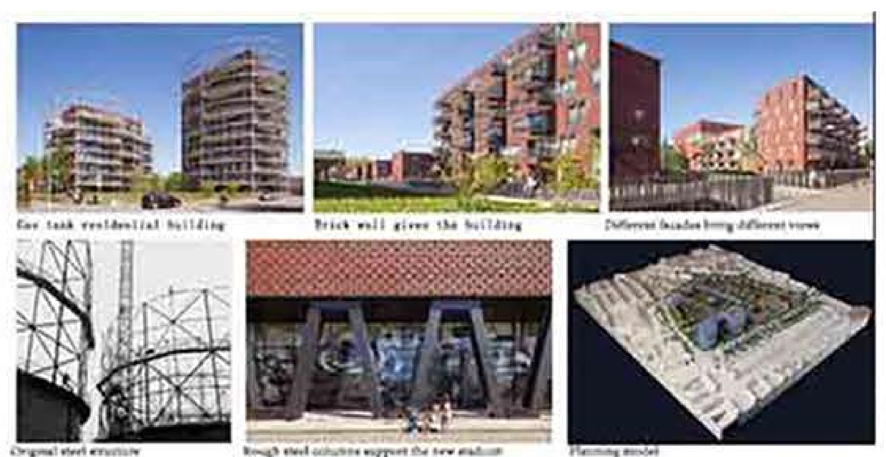
Fig 7 Old gas plant renovation - Villa Industria
