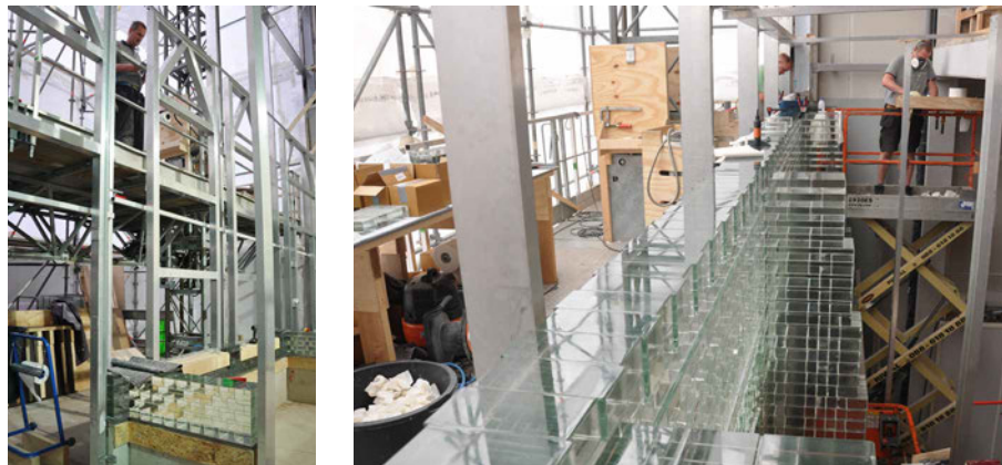
FIG. 6.9 Left: the installed aluminium place holders of the opening. Right: The mast climbing working platform and one of the three mobile elevated platforms.
