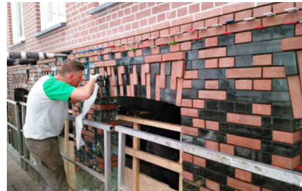
FIG. 6.16 The top connection is completely masked by the ceramic strips.
