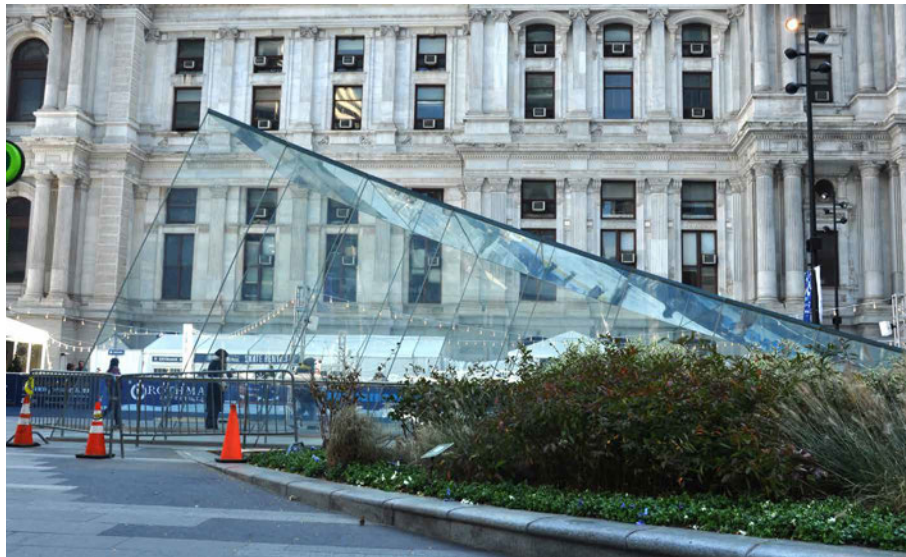
FIG. 2.3 Glass structure out of standard float panels up to 6 m in length by EOC Engineers in Philadelphia, USA.
