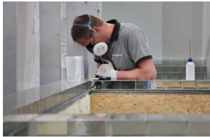
FIG. 6.15 Left: Sealing of the already bonded bricks. Right: the final, visual result achieved by the novel bonding method.
