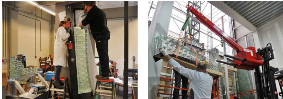
FIG. 6.17 Left: The special rotating fixture for the preassembly of the architraves. Right: The installation of the bonded architraves on site.
