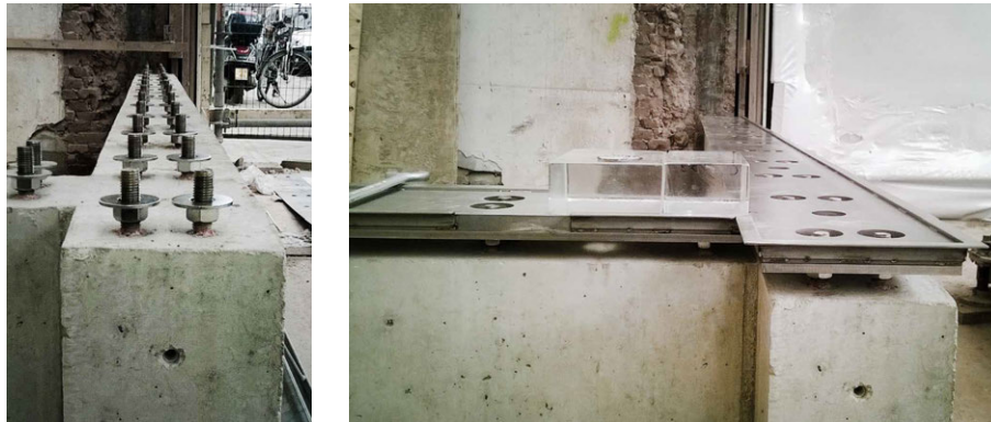
FIG. 6.10 On the left the bolts used for levelling the stainless steel plate, seen on the right.
