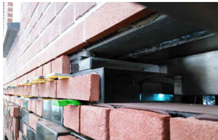
FIG. 6.16 The top connection is completely masked by the ceramic strips.
