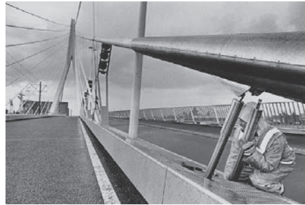
Fig. 1: Used new dampers to the Erasmus bridge to prevent vibrations. Photo: courtesy of TU Delft.
