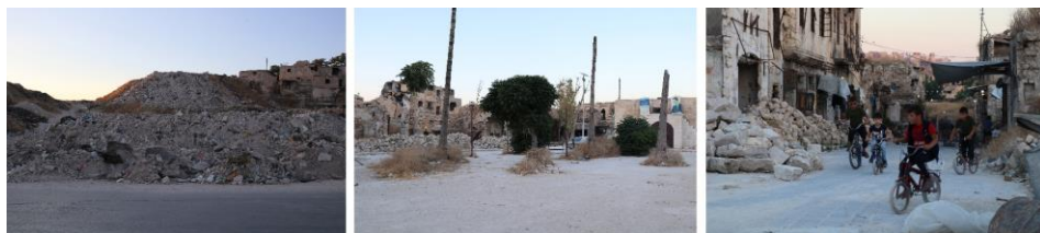
FIGURE 10: Accumulation of debris in Tallet Alsauda, sorting stones in Al-Hatab Square, sorting stones on-site; (left to right). Source: Totol Real Estate Title & Development in Aleppo, 2019
