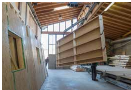
FIG. 8 SINFONIA project – panel production (source: Benedikter Architekten)
