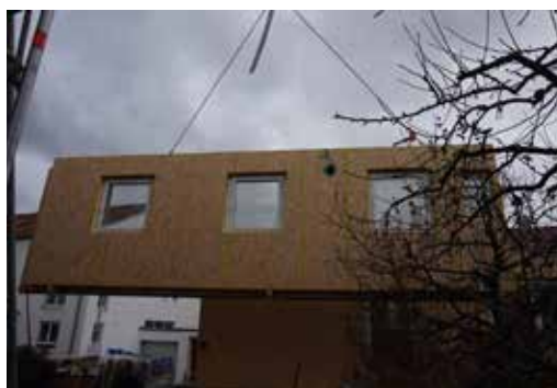
FIG. 4 iNSPIRe facade installation sample, internal side view (source: Gump & Maier)
