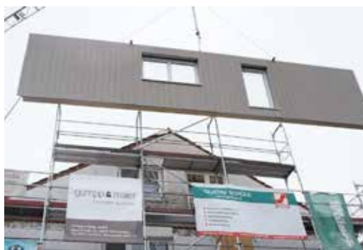
FIG. 3 iNSPIRe facade installation sample, external side view (source: Gump & Maier)
