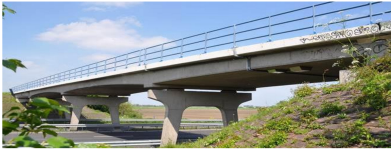
Figure 3. Example of a common four-span plate bridge type in the Netherlands: Bridge Zijlweg of the highway A59 in the province Brabant.
