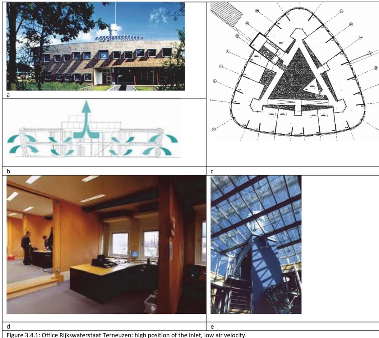
Figure 3.4.1: Office Rijkswaterstaat Terneuzen: high position of the inlet, low air velocity.
