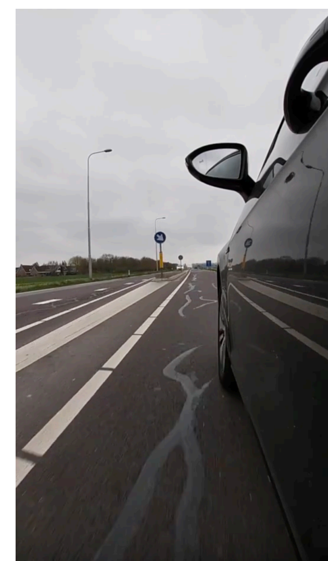
Asphalt repair patches
