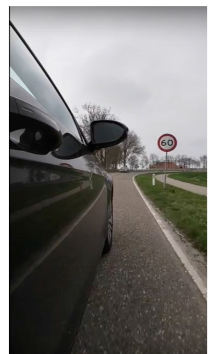
Speed reduction limit placed too late before a curve
