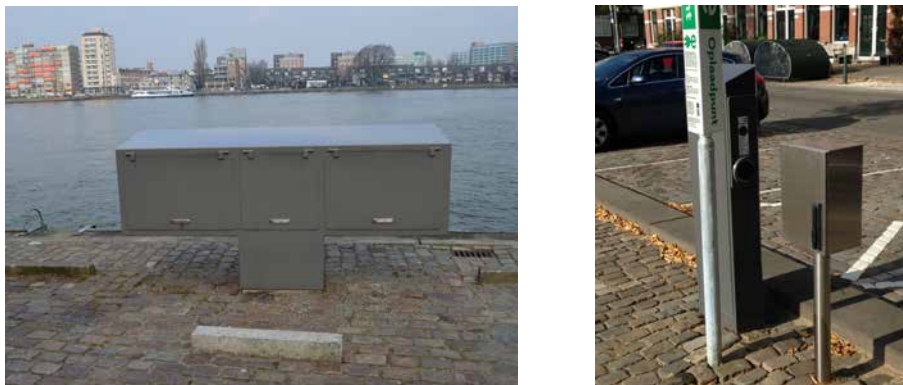
FIGURE 4.15 Elevated shore power supply facility in Dordrecht, The Netherlands (left) and flood protected power distribution station at the Noorderiland, The Netherlands. Photos by author.
