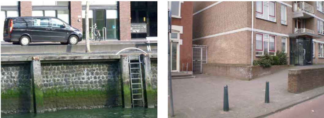
FIGURE 4.9 Left picture: land elevation at an urban development of the former port area in Rotterdam (Müllerpier). Note that the land elevation keeps a distance from the bulkhead to avoid structural integrity problems of the historical quay construction. Middle picture: elevation of an infill building (Feijenoord, Rotterdam). Photos by author.
