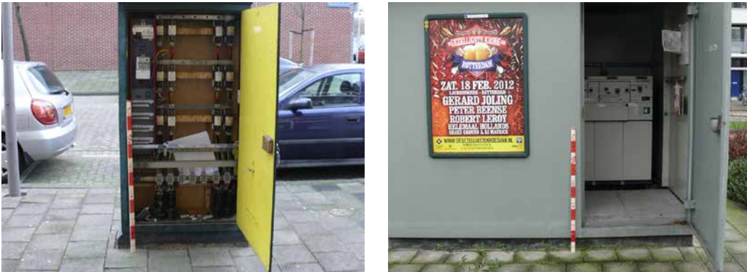
FIGURE 5.3 Typical low voltage (left pictures) and medium voltage distribution stations (right picture) at Rotterdam. Critical threshold of these cabinets is an inundation that reaches depths of 30 and 50 cm respectively. Photos: Robert de Kort (2012).
