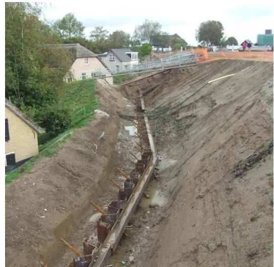
Figure 1: Installation of discontinuous sheet pile wall as reinforcement of Lekdijk Krimpenerwaard
