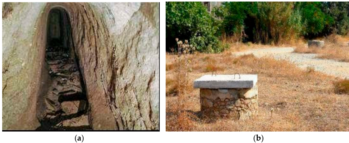
Figure 12. Roman underground aqueduct in the Aegean island of Rhodes, Greece: (a) part of the underground tunnel; (b) aligned shafts at the ground surface (photos by A. N. Angelakis).
