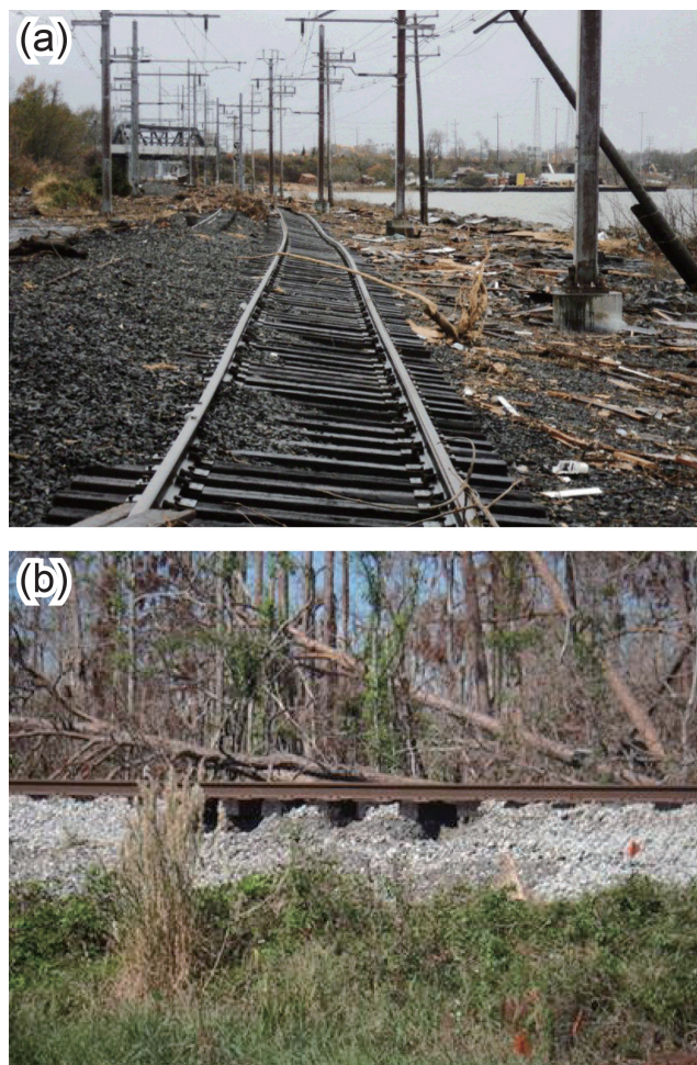
Figure 1. Railway ballast scour failures: (a) New Jersey Transit tracks in New Jersey, USA, after Hurricane Sandy in 2012; (b) CSX railroad tracks in Mississippi, USA, after Hurricane Katrina in 2005 (photo credits: New Jersey Transit, a).
