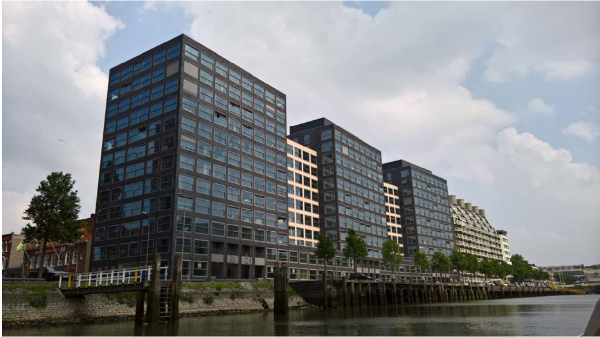
Figure 4.2. Case study 'De Admiraliteit' after completion (source: Remøy).
