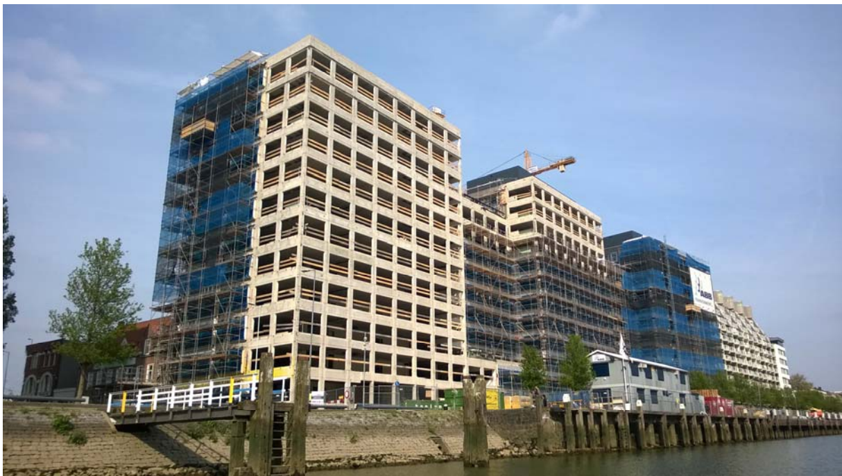
Figure 4.1. Case study 'De Admiraliteit' during construction (source: Remø).
