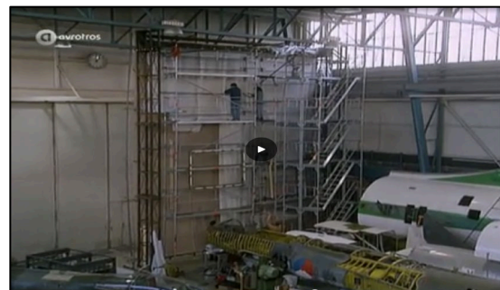
Figure 1. (b) Film still of the on-scale test setup to work out the relining process in the aircraft hall of the faculty of Aerospace Engineering of TU Delft in the beginning of 1990. NPO Closeup 1996. https://www.npostart.nl/close-up/11-07-2015/AT_2037854
