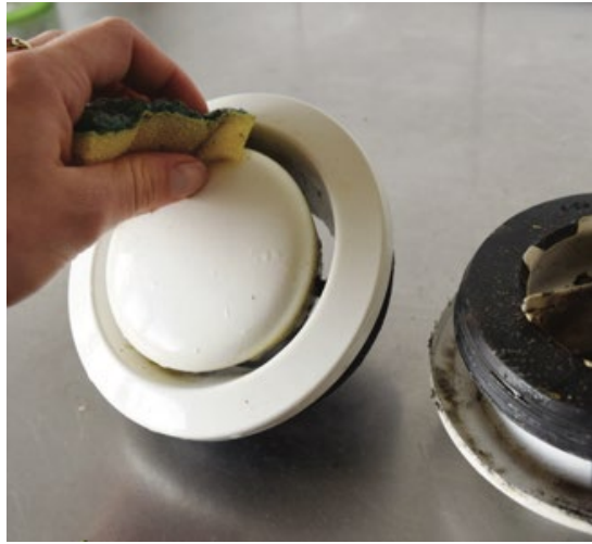
Figure 11 Residents are expected to clean the valves. But cleaning them without adjusting configuration or mixing up valves is a challenge
