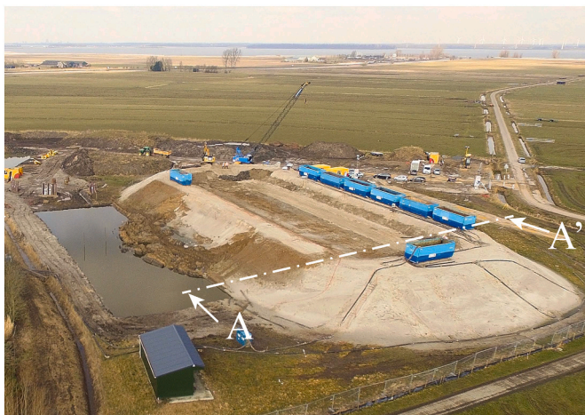
Fig. 7. Aerial photo of the Eemdijk ring-shaped test dike, with slope instability of the conventional (ground) dike (left). The test dike with sheet pile, is located on the right side. Image courtesy of Eric Feijten/NOS (Feijten, 2018).
