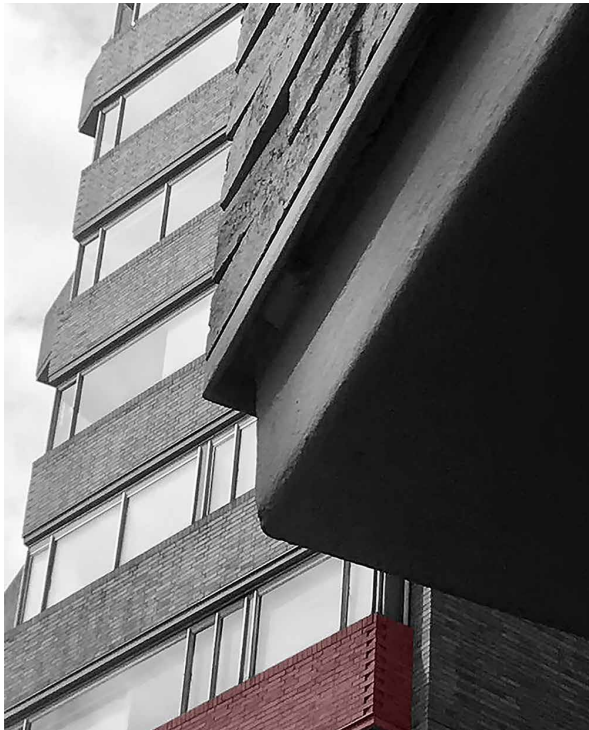
FIG. 9 Photograph of Torres del Parque light façade wall that works as a buttress, 1970. (Photograph by Faculty of Architecture & Design, Universidad de los Andes).
