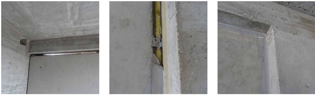
FIG. 7 Sealing joints of panel and load-bearing structure
