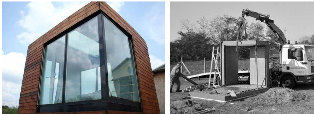
FIG. 5 Water House 1.0 completed (left) and during construction assembly (right)
