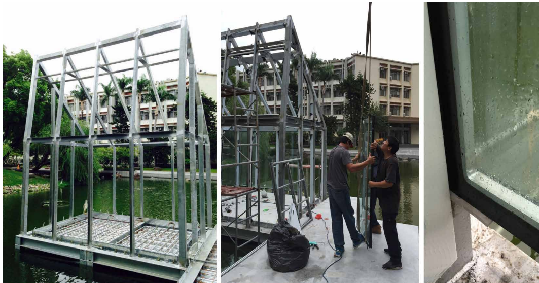
FIG. 9 Water House 2.0 during construction, showing the steel frame (left), positioning the panels (middle), and establishing the maintenance zone between floor and panel (right)
