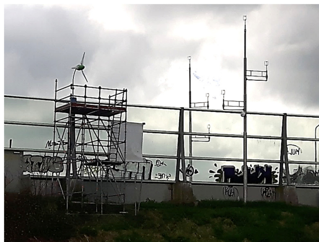
Figure 7. Micro wind turbine integrated on noise barrier field experiment. The 6 sonic anemometers are visible on the right located on two masts on three heights. The scaffolding behind the barrier is for access purposes and does not influence the incoming flow over the barrier.
