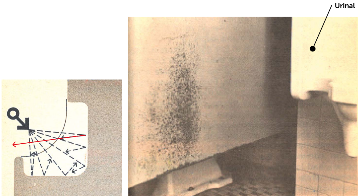
Figure 6.11a. The stream of urine (red arrow) causes backsplash on the wall (Kira 1976, 416)
