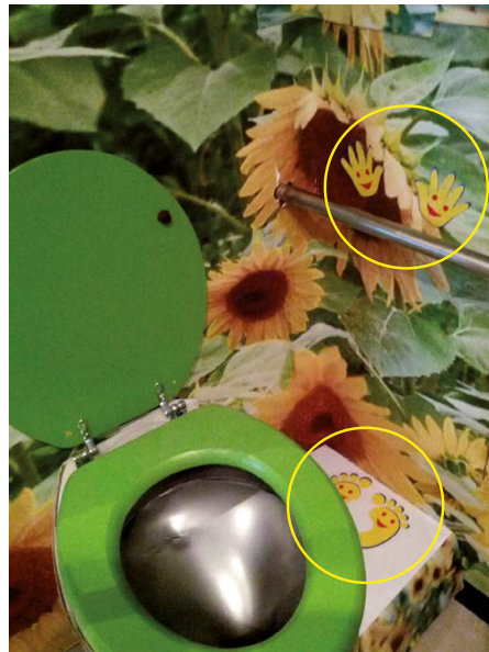
Figure 8.25b Children's platform at a height of 140 cm from the ground; sit-toilet with (happy) feet and hands above support bar
