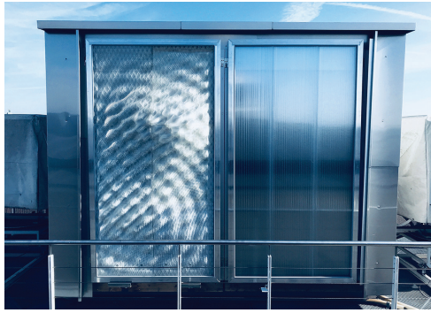
FIG. 16 Final Prototype of 3D Printed Future Façade
