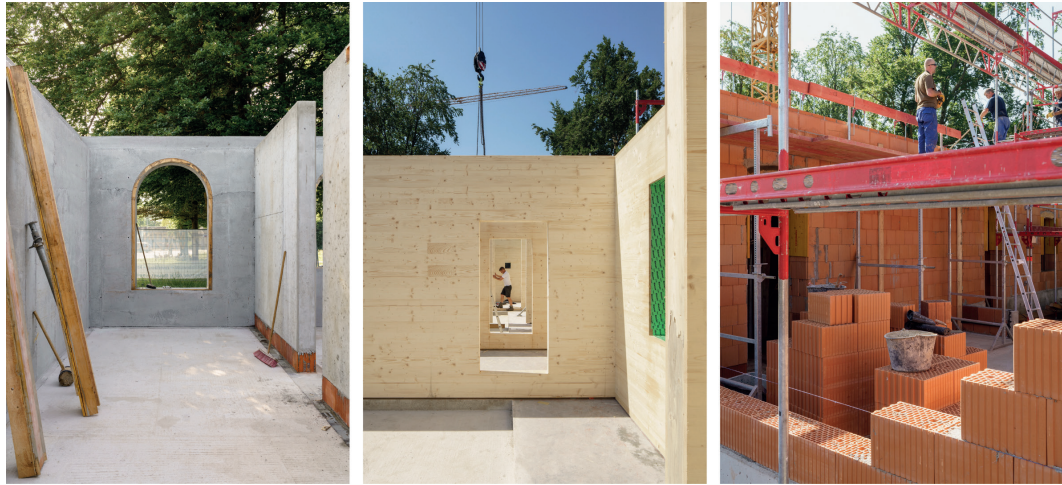
FIG. 14 The "Simply Build" research buildings in infra-light concrete, massive timber and masonry construction; Bad Aibling, Germany; @sebastianschels
