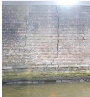
E. Tapered Crack
