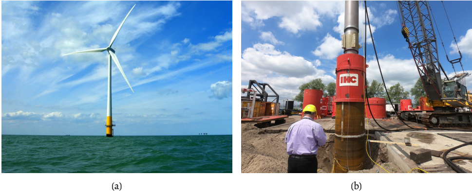
Figure 1.1: (a) Wind turbine in the Kentish Flats Offshore Wind Farm. Copyright 2008 by Phil Hollman. (b) Hydraulic impact hammer (IHC-IQIP S350) employed in an onshore monopile installation.
