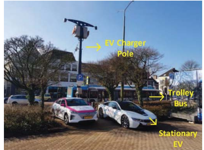
Fig. 1: Stationary EV charging by co-utilizing the trolley-bus network [10].
