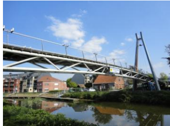
Figure 1. The footbridge in Ninove, Belgium.
