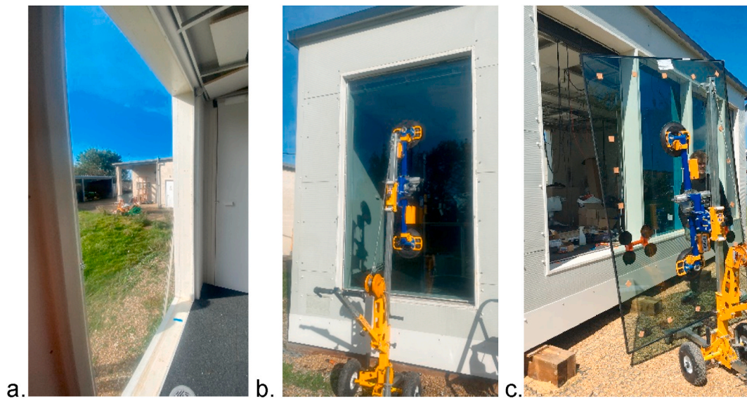
Fig. 5. Reconfigurable facade (a). Reconfigurable wood frame. (b). External view of the façade panel with the glass lifter before the removal; and (c) Removal of the glass panel with the glass lifter.
