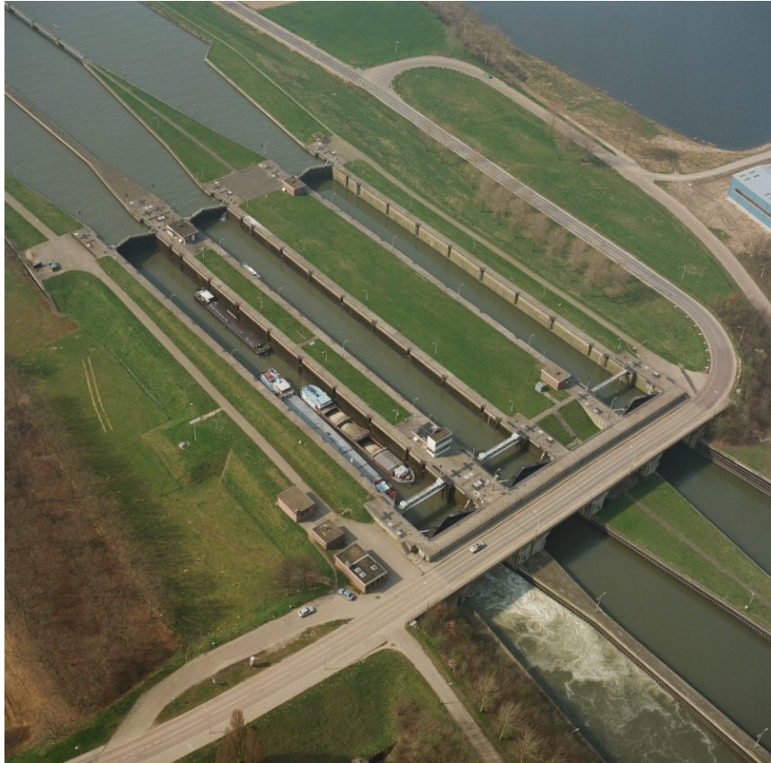
Figure 3.2: Locks at Lith for commercial traffic at the Maas river ( image by https://beeldbank.rws.nl , Rijkswaterstaat, by: Bart van Eyck).
