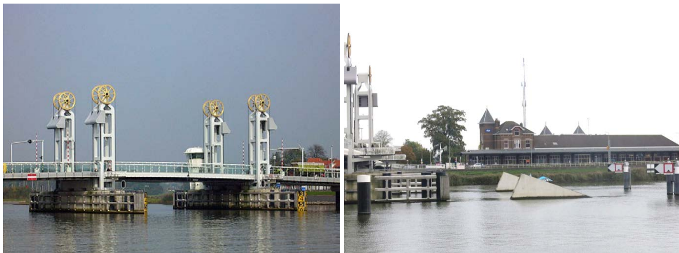
Figure 3.31: Left: City Bridge, Kampen (NL), without concrete ramps (Kampen stadsbrug hefgedeelte by Arend041 is licenced under CC0 1.0); right: with concrete ramps (courtesy Yttje Feddes is licenced under CC BY-NC-SA 4.0).
