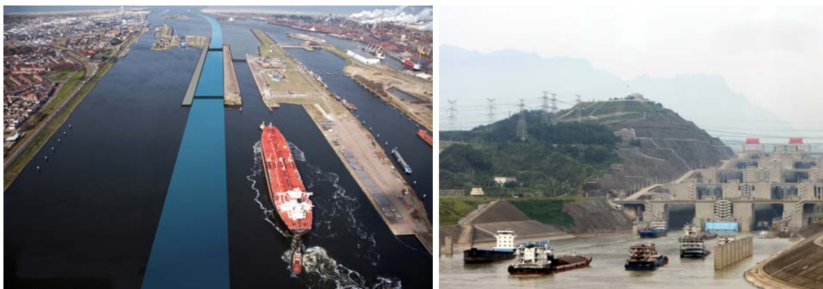
Figure 3.1: Multiple-lock systems. Left: Sea Locks (major lock as projected), IJmuiden, Netherlands ( https://beeldbank.rws.nl , Rijkswaterstaat, by: Harry van Reeken); right: Three Gorges Project, China (Three Gorges Locks by RThiele is licenced under CC BY-SA 3.0).
