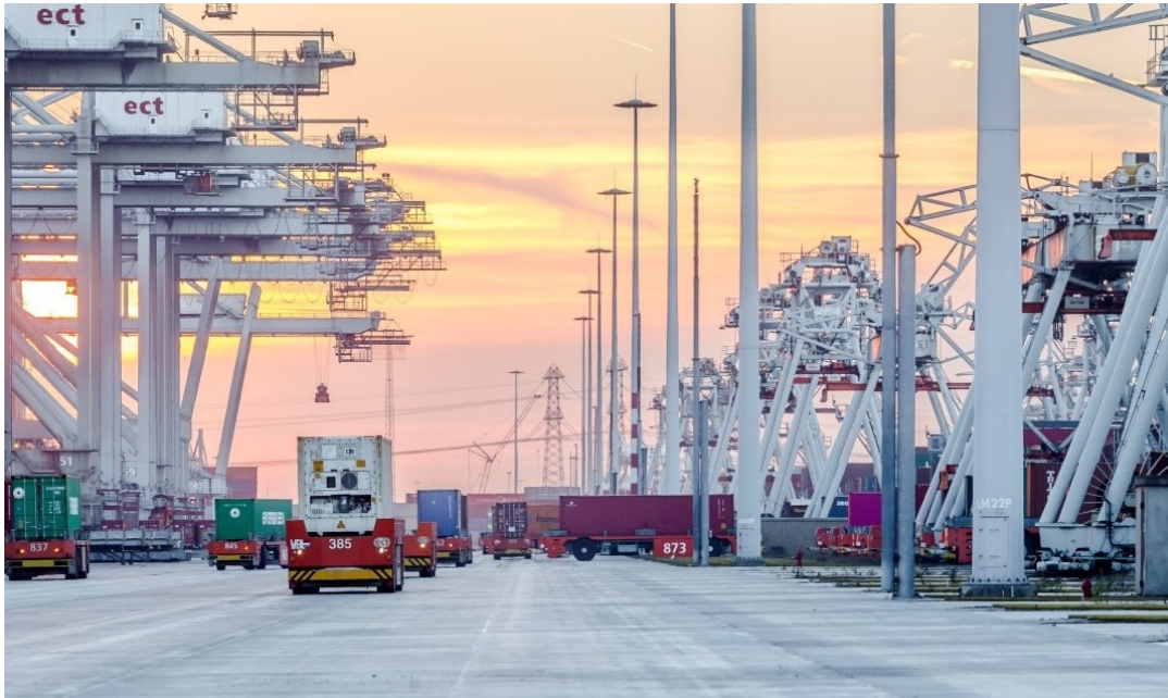
Figure 4.24: Automated Stacking Cranes (ASCs) (by ECT is licensed under CC BY-NC-SA 4.0).
