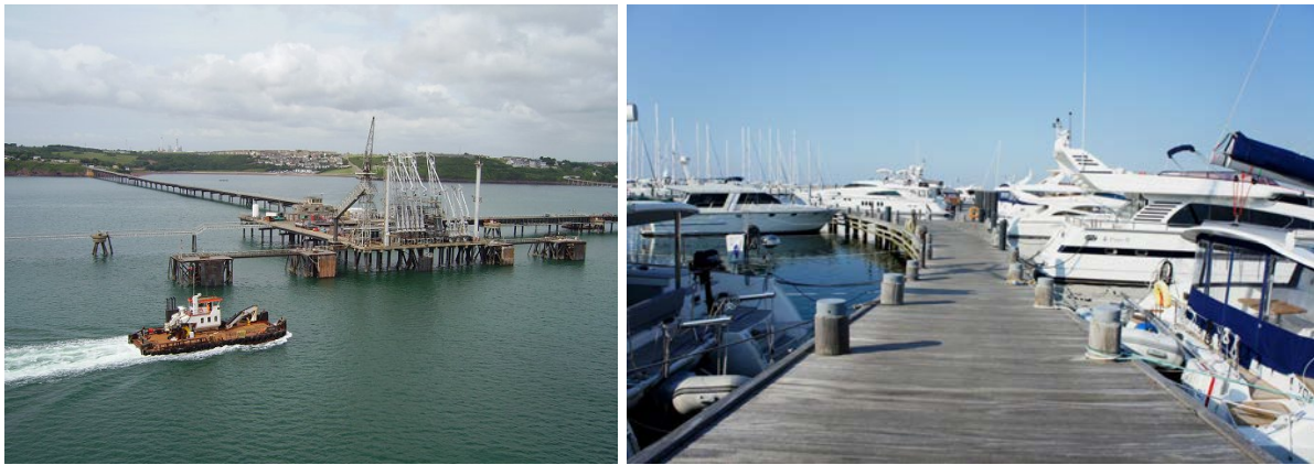
Figure 1.20: Left: Oil jetty, Total refinery, Milford Haven (by Richard Webb is licenced under CC BY-SA 2.0); right: Marina jetty (by pxhere.com is licenced under CC0 1.0).
