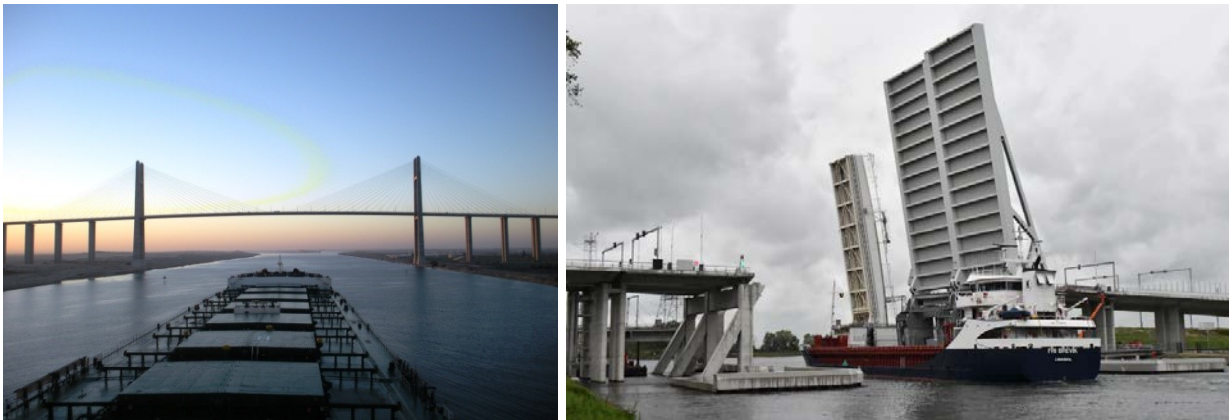
Figure 1.25: Left: Fixed bridge across the Suez Canal (by Aashay Baindur is licenced under CC BY-SA 3.0); right: Movable bascule bridge (by Tvx1 is licenced under CC BY-SA 4.0).
