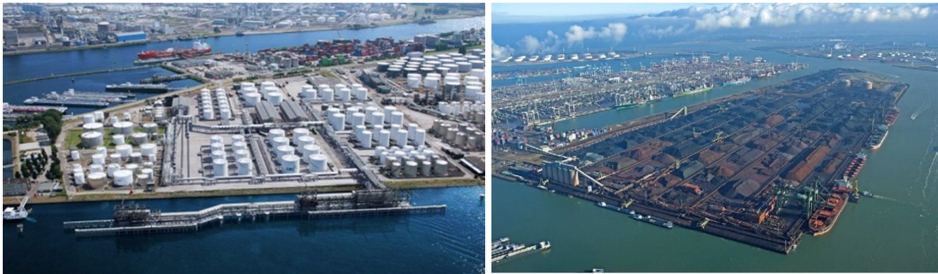
Figure 1.13: Left: Liquid bulk chemicals terminal, Rotterdam (by Royal HaskoningDHV is licenced under CC BY-NC-SA 4.0); right: dry bulk terminal, Rotterdam ( PIANC, 2019b ).
