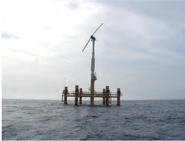
Figure 1.1: World's first floating wind turbine<sup>6</sup>.
