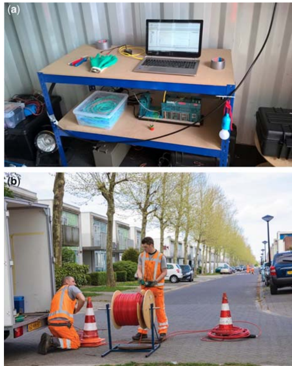
Figure 3.51 (a) DTS measuring computer, (b) Installation of a DTS cable. Source: courtesy Rémy Schilperoort (Partners4UrbanWater).
