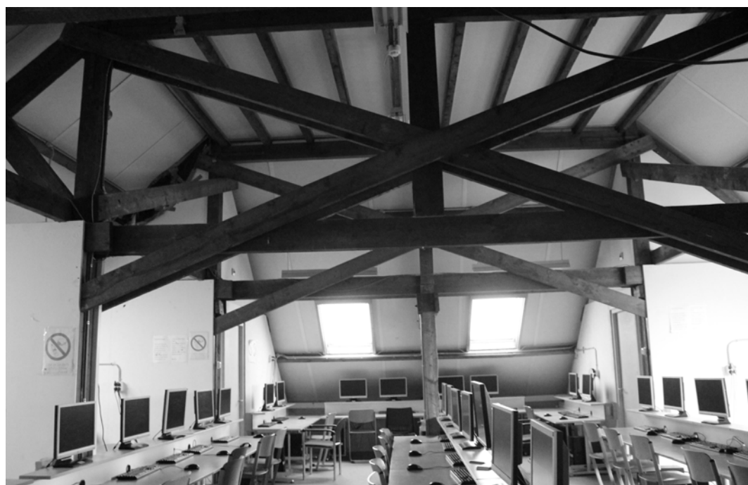
Timber roof construction
