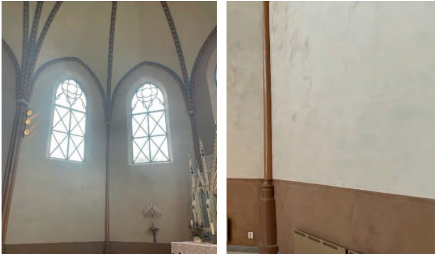
Figure 5: The two walls that have been plastered with hemp-lime in the choir. After two years there are no signs at all of salts on the surface. Only the normal liveliness of the lime wash gives the surface its expression.
