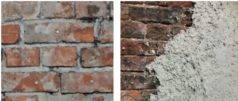
Figure 3: Stainless-steel wire (left) and chicken wire (right) acted as a reinforcing and plaster-bearing system. The hemp-lime had been applied here in a thickness of 10-30 mm directly against the brick wall.
