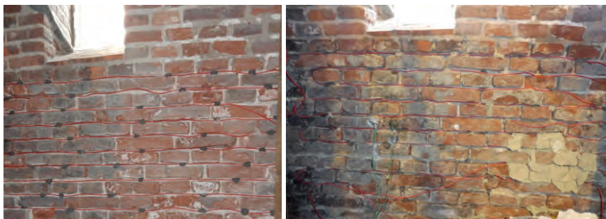
Figure 8: Location C (heated) before desalination (left) and after desalination (right): no further damage due to desalination is observed.
