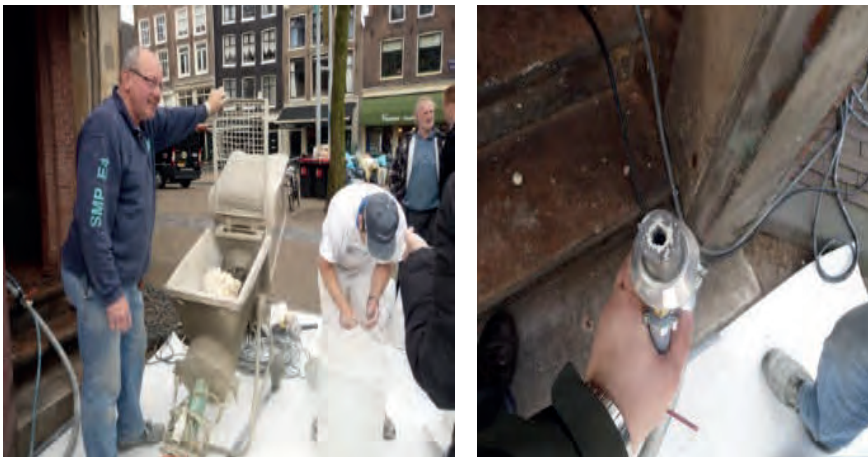
Figure 2: Using a stucco sprayer.
