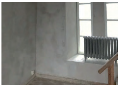
Figure 7: Lime plaster finish of NHL3.5.
