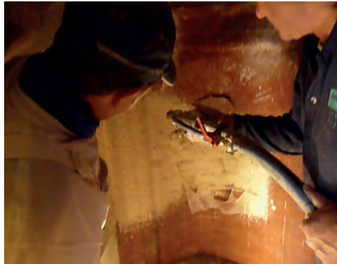
Figure 3: Spraying of the poultice.
