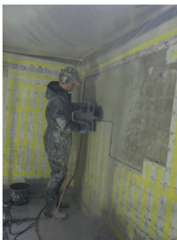
Figure 3: Removing the tiles using a diamond saw.
