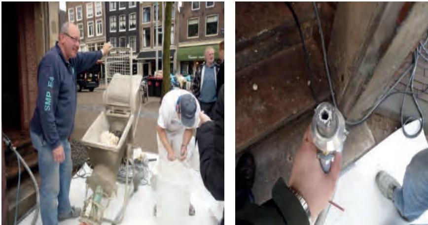
Figure 2: Using a stucco sprayer.
