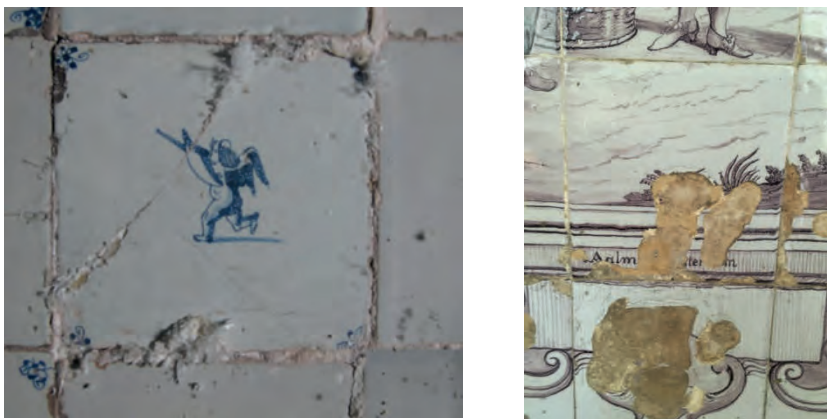
Figure 1: Salt efflorescence on the sides of a tile and along a breakage (left); blistering of the glaze (right).
