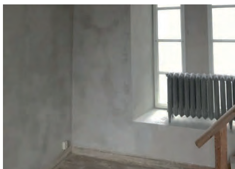
Figure 7: Lime plaster finish of NHL3.5.
