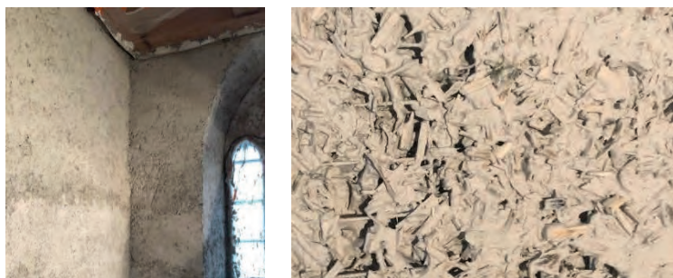
Figure 6: Hemp-lime as an insulating base layer at Örgryte New Church.
