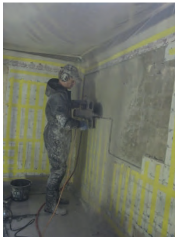
Figure 3: Removing the tiles using a diamond saw.
